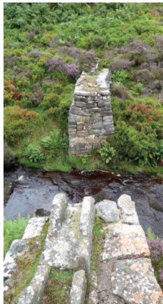
Piers and stone channel, Bonfield Ghyll
