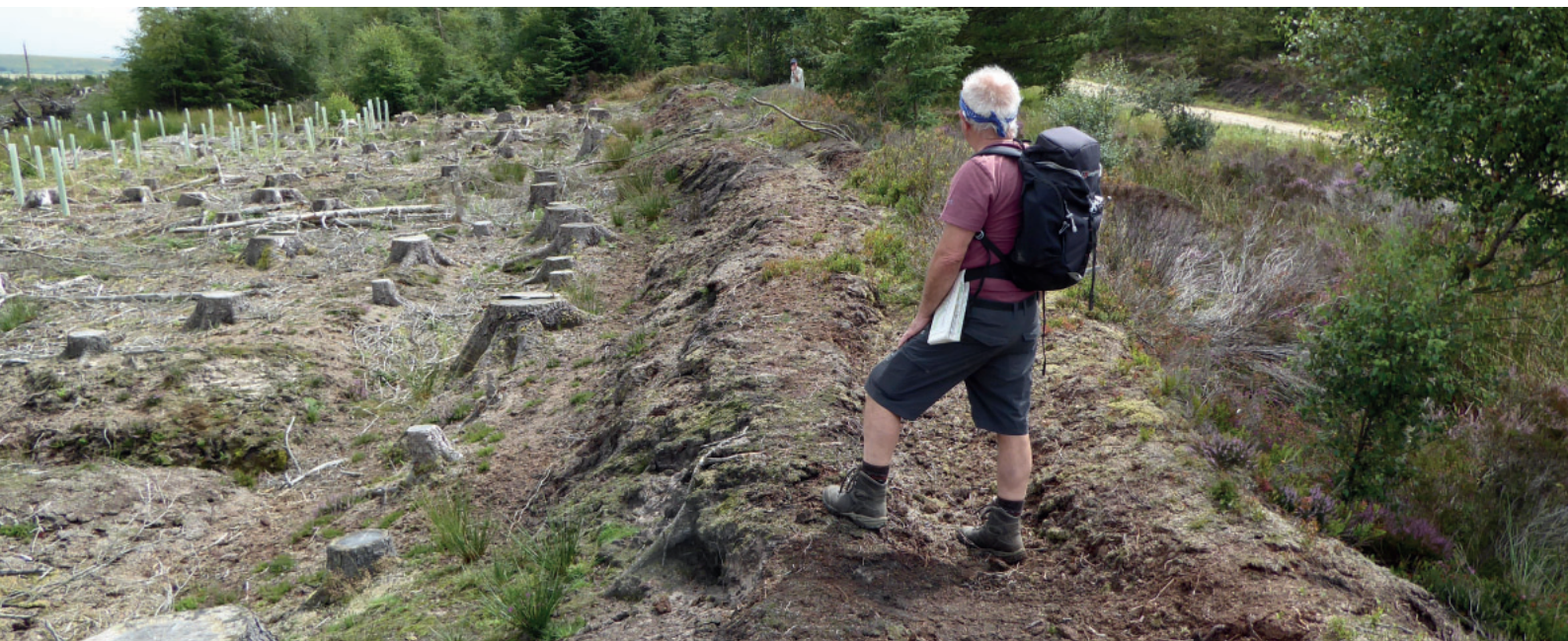
'Floating' embankment, Roppa
